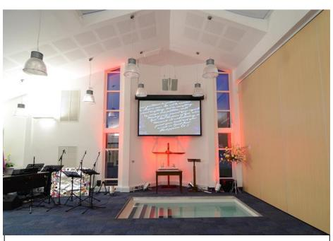
Dual motor winch screen allows the casing to rise close to the ceiling. A central Electrovoice ZX1i speaker cluster ensures total room coverage and with a matching subwoofer, provides exceptional full range music reproduction.
