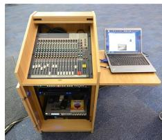
Bespoke rack contains all tactile audio-visual equipment with folding side laptop shelf. Adjacent picture shows platform-facing LCD display
